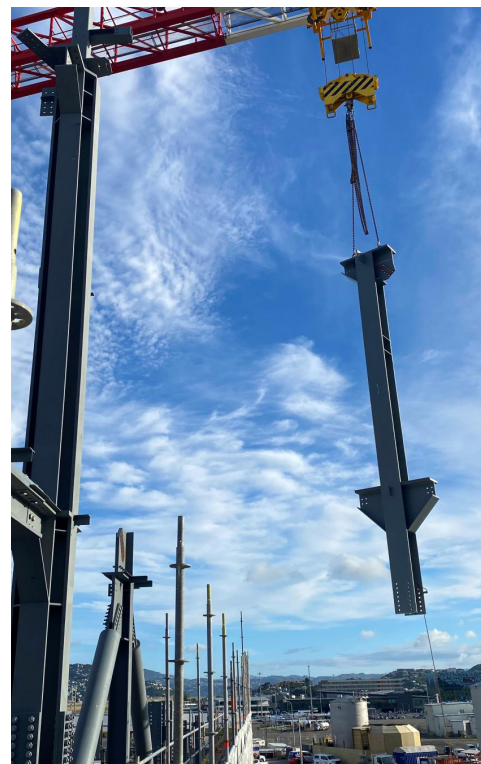
Beams and columns being lifted
