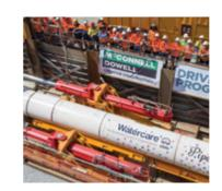
Adopting new trenchless technology to install a world record 2021 m long, 1220 mm diameter pipe without the disruption and environmental impact of a trench.
